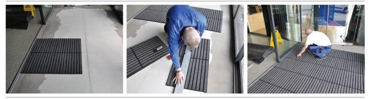
Matrix and Concourse Tiles require no permanent bonding they are designed to be loose laid. They require butting tightly in all directions. Leave no more than a 3 mm gap around the perimeter of the matwell as the modules do not expand.
